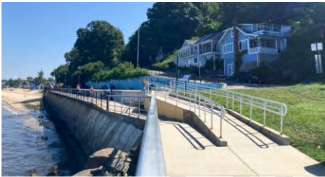
Accessible ramp at Cliff Way
