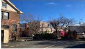
REAR PARKING LOT
