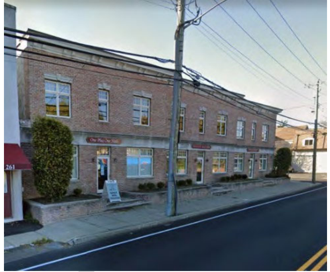
Mixed-use building on Glen Cove Avenue
