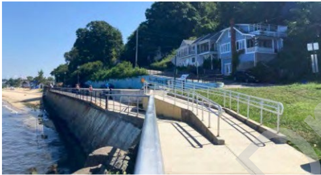
Accessible ramp at Cliff Way
