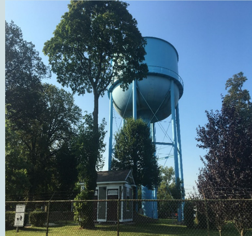
Sea Cliff water tower
