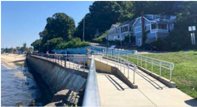
Accessible ramp at Cliff Way
