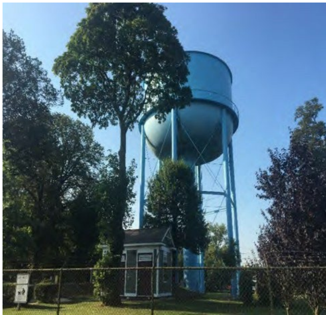
Source: Water System Valuation and Feasibility Study Sea Cliff Water Tower
